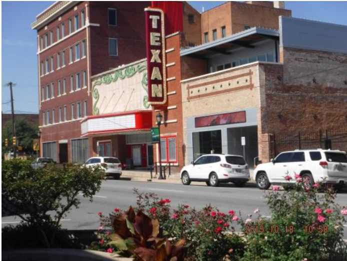
Downtown Greenville and the newly renovated Texan Theater.
